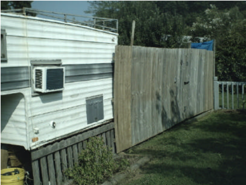
Outside of area showing A/C and camper
