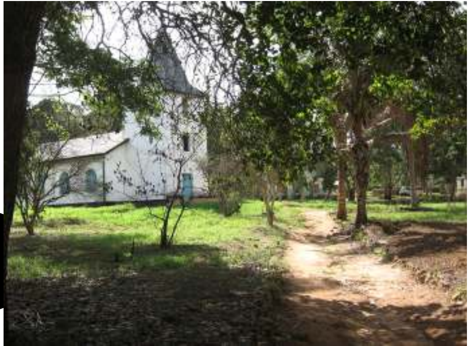
The Maneromango church. The building fell apart once and this one was rebuilt as a replica of the old.
